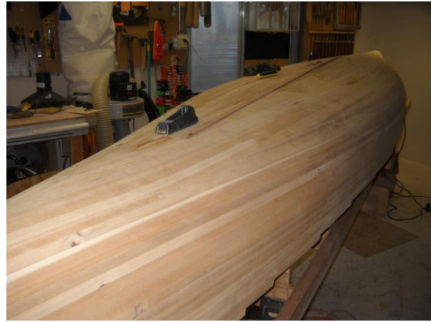
Canoe currently under construction
